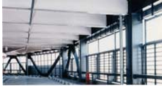
Photo. 8. Steel Frame of Sen City Car Plaza
