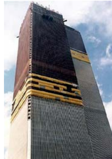
Photo 1. WTC under construction
