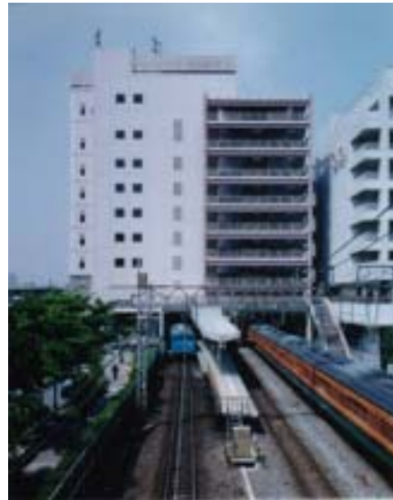
Photo. 10. Steel Frame of Sen City Car Plaza
