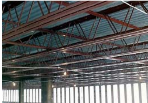
Photo 3. Floor truss (before protected)
