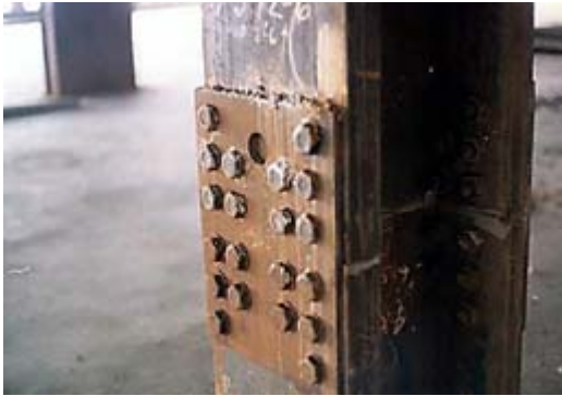
Photo 2. Core column (ultra-jumbo H-shape)
