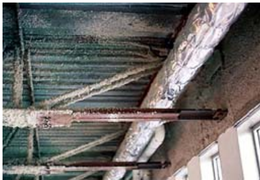
Photo 4. Fire Protection of floor truss
