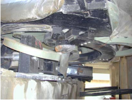
Figure 6- Damage to an EDU, shear key and a pot bearing
