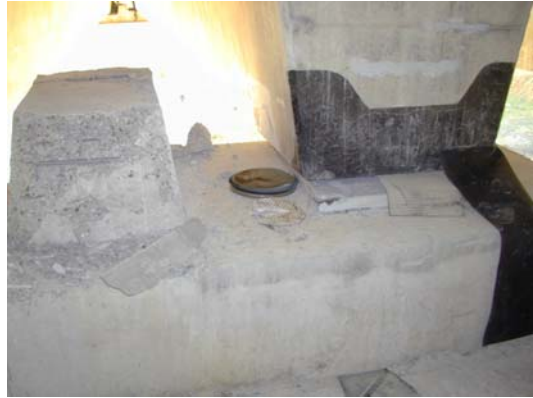
Figure 6- Damage to an EDU, shear key and a pot bearing
