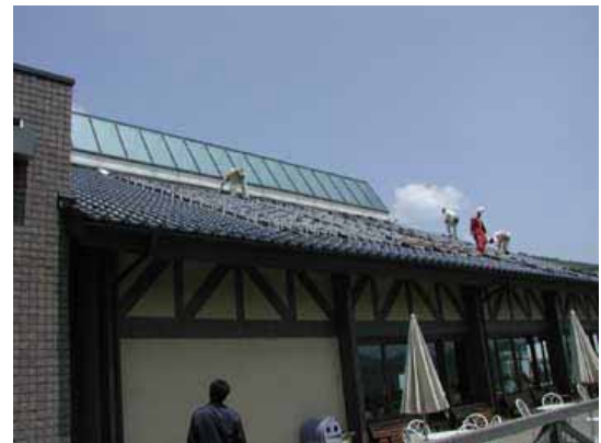
Photo 4 Repair work for roof tiles
