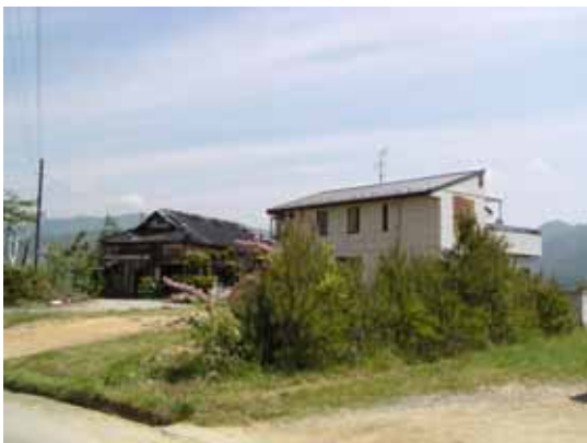
Photo 11 Two "severe-damage" residences
