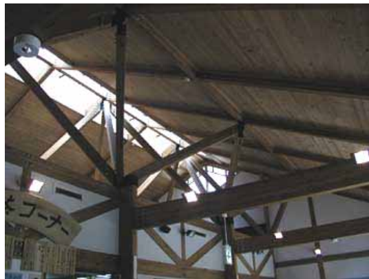
Photo 3 Truss construction using large section members
