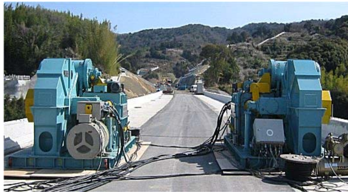
Photo 1 Installation of the exciter on the road surface
