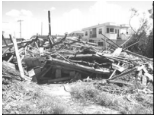
Photo.7 Collapsed Old Timber House (Miyako Island)
