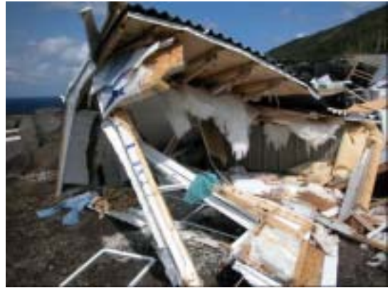
Photo.12 Collapsed Trailer House Standing near Cliff of Seashore (Hachijo Island)
