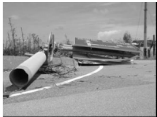
Photo.17 Collapsed Traffic Sign (Miyako Island)
