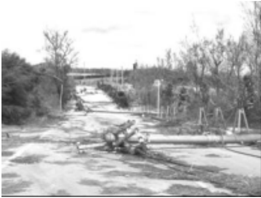
Photo.18 Row of Collapsed Telegraph Poles (Miyako Island)
