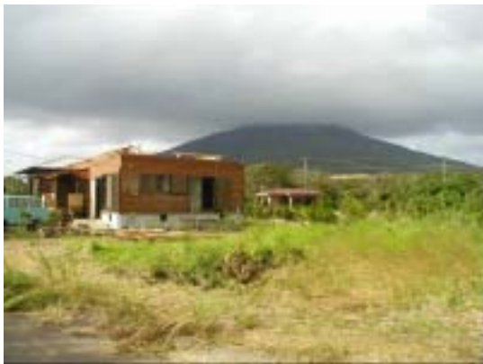
Photo.10 Collapsed Roof Frame of Timber House (Hachijo Island)
