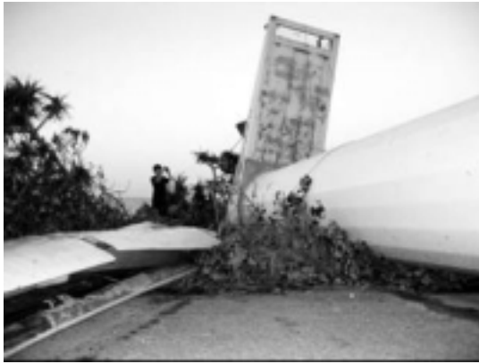
Photo.13 Broken Blades and Nasal of Wind Turbine Generator System (Miyako Island)
