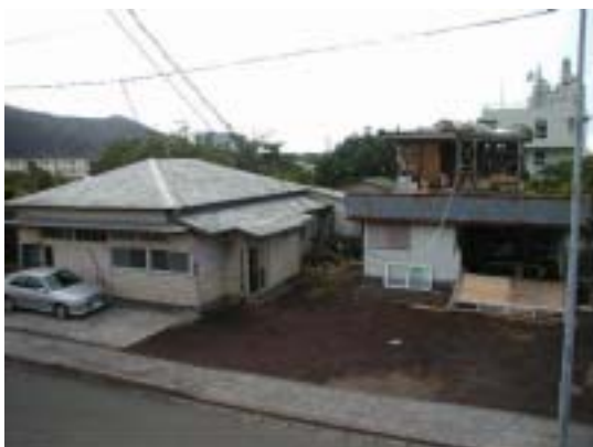
Photo.11 Marked Contrast between Damaged and Non-damaged Houses (Hachijo Island)
