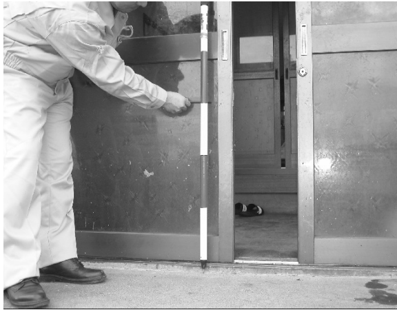
Picture 3. Inundation Mark at a House in the Interior Area of the Tokachi Port
