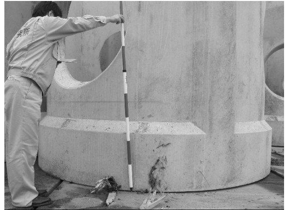
Picture 6. Inundation Sign on the Blocks in the Bending Part of the Otsu Fishery Port
