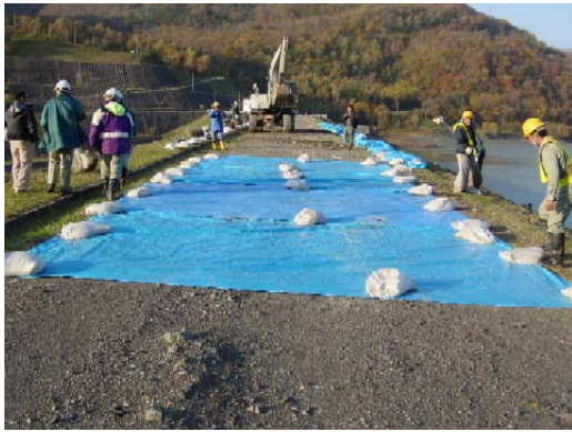
Photograph 7 Protection of Cracks at Crest (Takami Dam)
