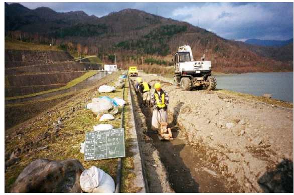
Photograph 8 Repair Work of Crack Locations (View of Excavation) (Takami Dam)
