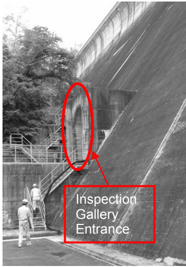
Photograph 3 Inspection Gallery Entrance on Right Bank Abutment (Tase Dam)
