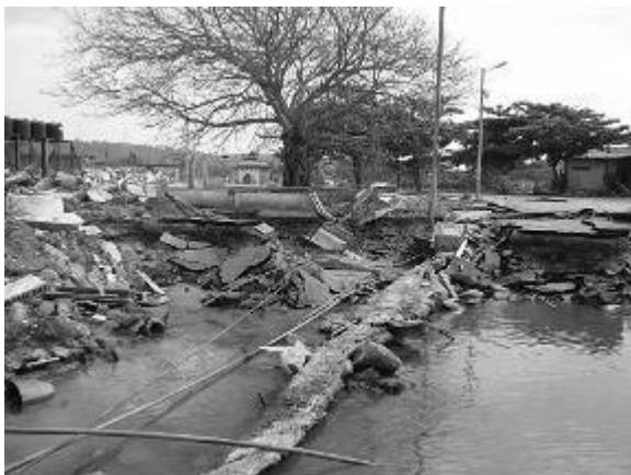
Photo 4: Damage of quay wall.
