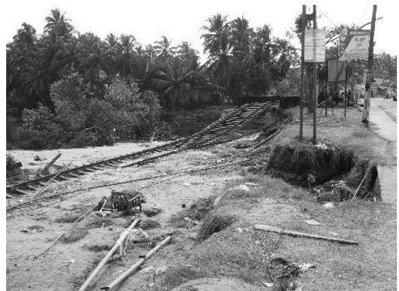
Photo 6: Damaged railway by erosion.
