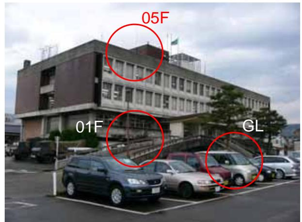
Photo 4 Locations of seismometer at OJC
