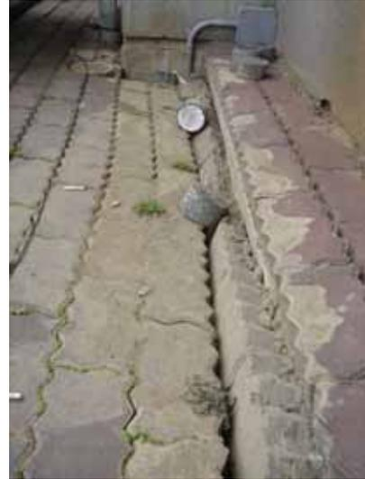
Photo 2 The ground deformation by subsidence (OJC)
