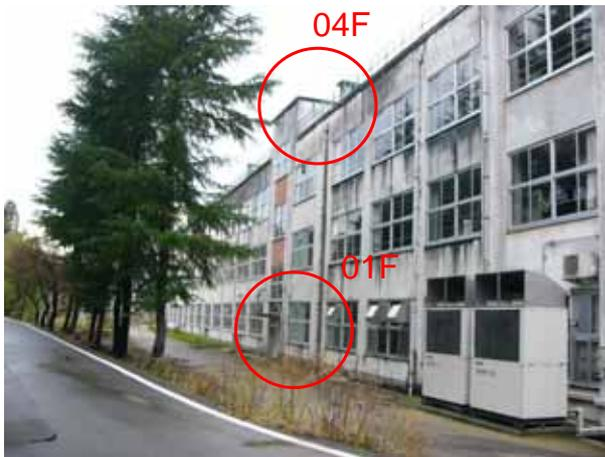
Photo 3 Locations of seismometer at OJP
