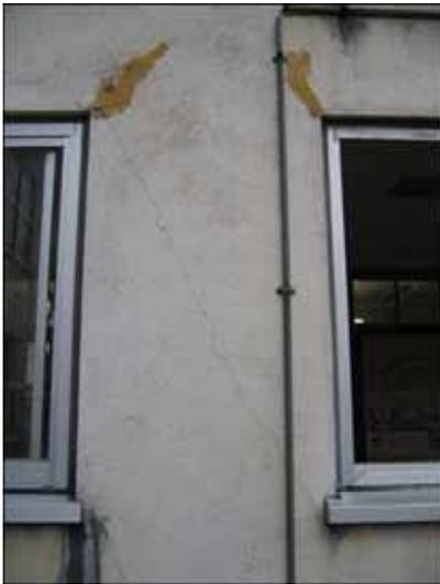
Photo 1 Shear crack on column (OJP) [3]
