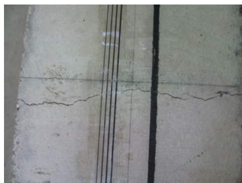
Figure 7 : Crack in this test specimen and electrically conductive materials after unloading
