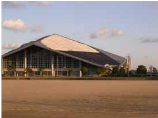
Fig.6 Failure of Public Gymnasium
