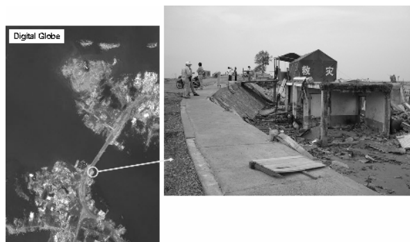
Picture 1 Reduction of tsunami damage by a road mound in Banda Aceh
