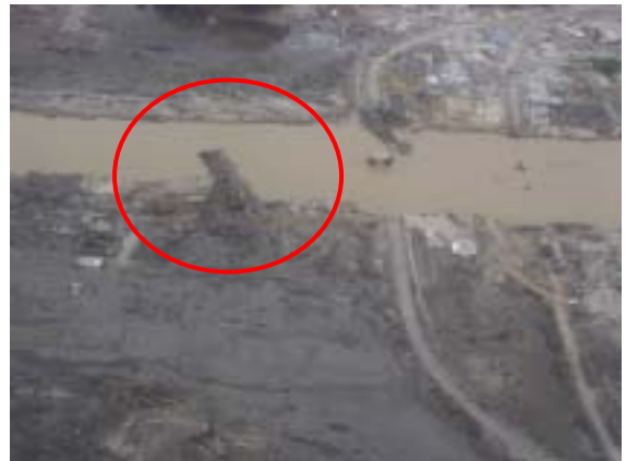
Photo 23 Washout of Truss Bridge (2)
