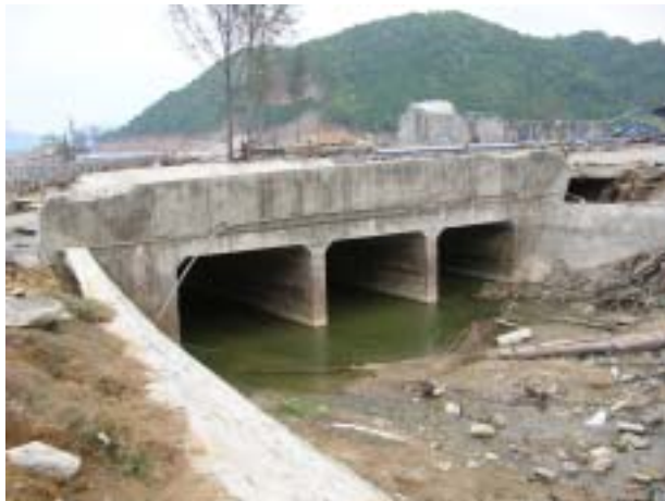
Photo 20 Concrete Box Culvert Bridge
