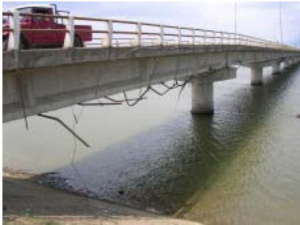
Photo 11 Undamaged Bridge by Tsunami
