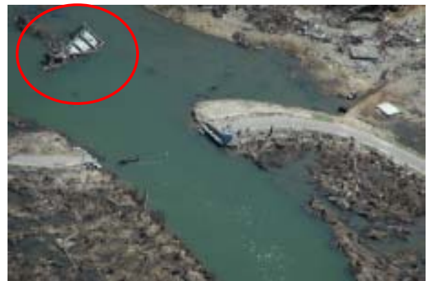
Photo 25 Washout of Truss Bridge (4)
