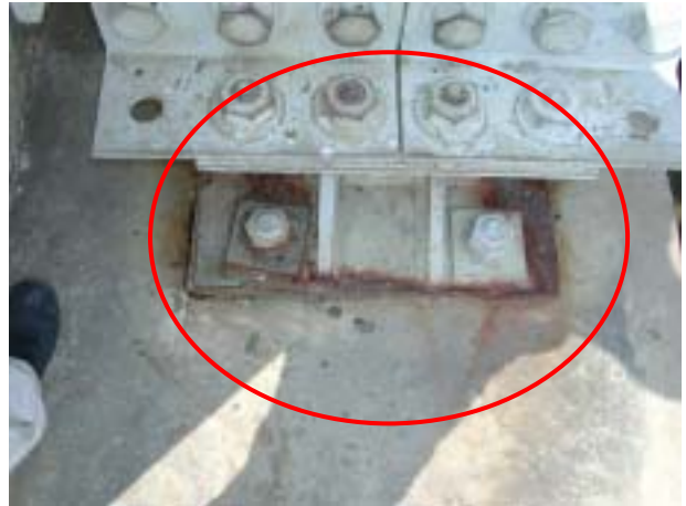
Photo 16 Steel Bearing Supports
