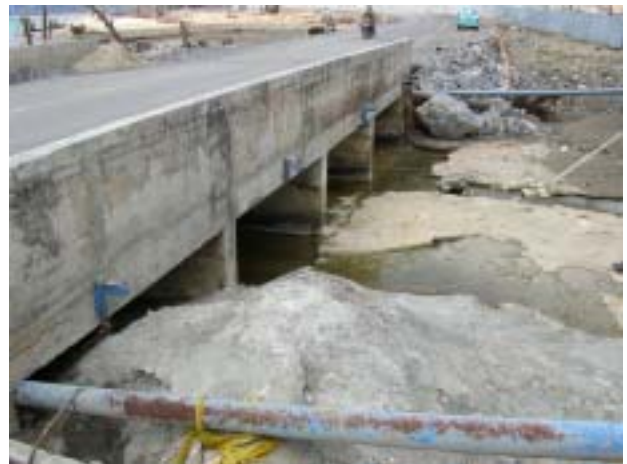
Photo 21 Concrete Box Culvert Bridge
