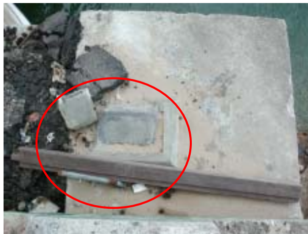
Photo 19 Bearing Support and Bolt to connect between Deck and Substructures
