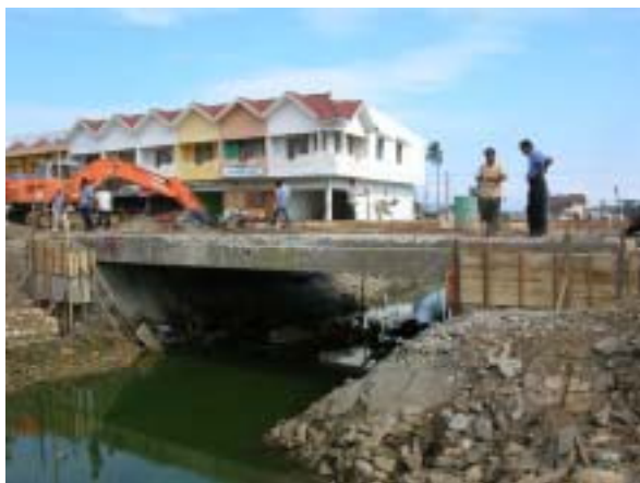
Photo 1 Repair of Washed-out Girder
