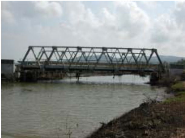
Photo 15 Steel Truss Bridge without Damage
