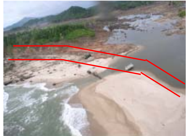
Photo 27 Erosion of Road and Coastline
