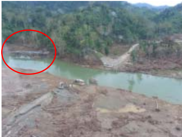
Photo 26 Washout of Truss Bridge (5)
