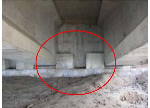
Photo 12 Concrete Block Shear Keys
