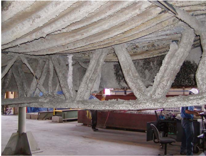
Figure 2. Buckled truss webs and bowed metal deck
