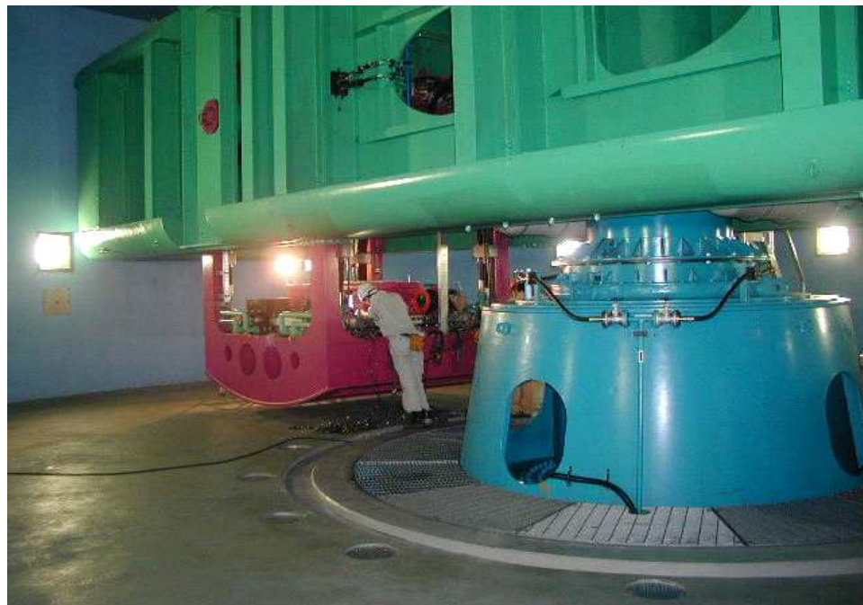
Figure 16: Centrifuge Facility at Obayashi Corporation, and Gravity Dam model
