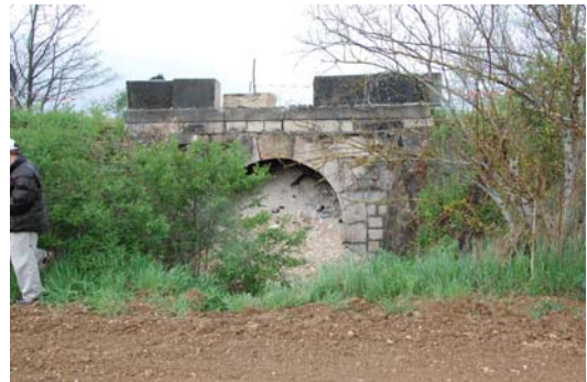
Photo 19 Emergency repair of a stone masonry arc culvert (SR261)
