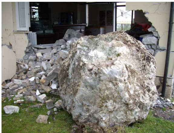
Photo 6 A 12 ton fallen rock with 1.9m long, 1.6m wide and 1.5m tall
