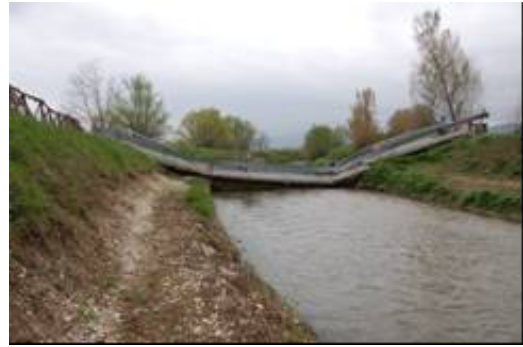
Photo 11 Collapse of a three span continuous bridge near Fossa Station
