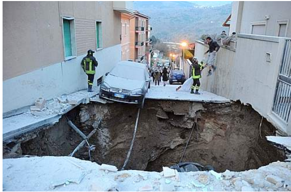
Photo 8 Sinkhole immediately after the earthquake (from Web page)
