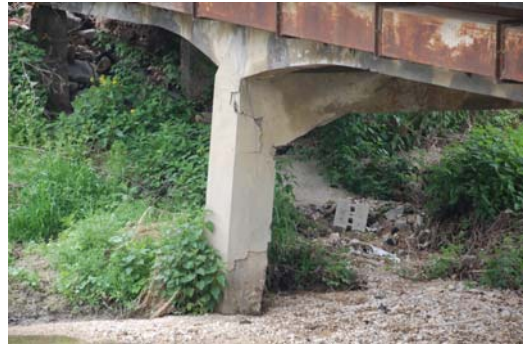
Photo 18 Damage of a frame reinforced concrete pier
