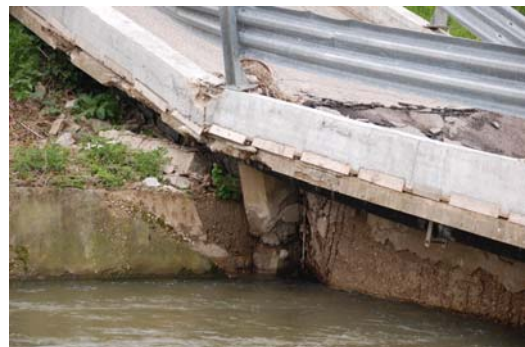
Photo 13 Damage of pile-bent pier
