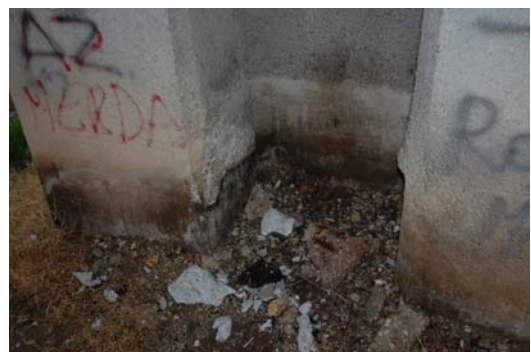
Photo 24 Spalling of a part of covering concrete
