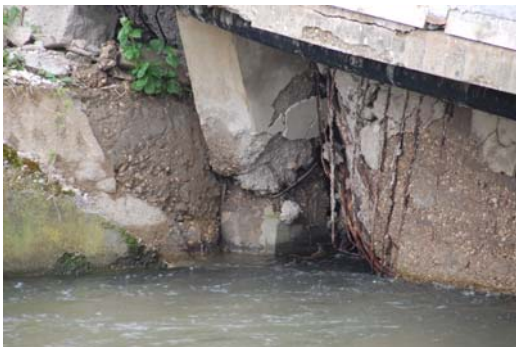
Photo 16 Failure of a pile-bent pier
