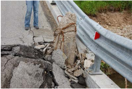
Photo 15 Top of a pile-bent pier
