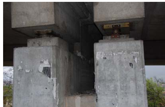
Photo 25 Damage of a shear connector
