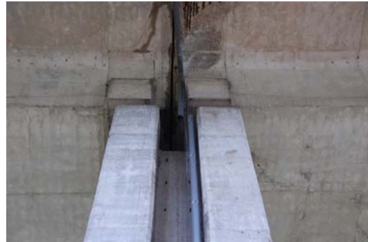
Photo 23 Residual drift of two bridges in the longitudinal direction
