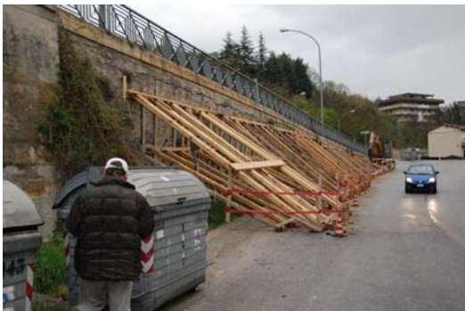
Photo 27 Emergent repairing of damaged embankment
