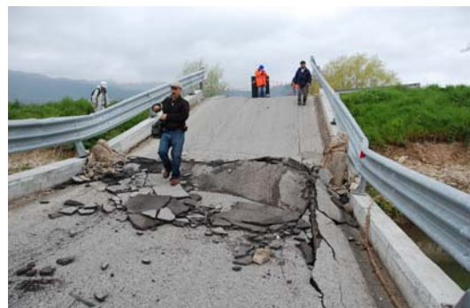
Photo 14 Pile-bent piers which punching sheared the deck slab
