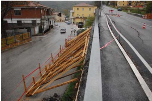
Photo 26 Subsidence of a road embankment at the intersection of Route SS17 and Route SR615
