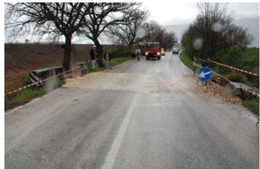
Photo 20 Road temporarily repaired by filling crashed limestone
