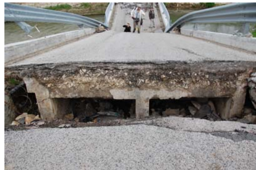
Photo 12 Section of the fallen deck
