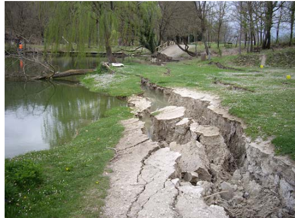
Photo 4 Separated blocks due to lateral spreading
