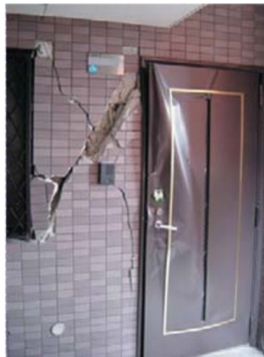
Photo 2 Crack damage of nonstructural wall of corridor of a condominium by the West-Off Fukuoka Earthquake in 2005
