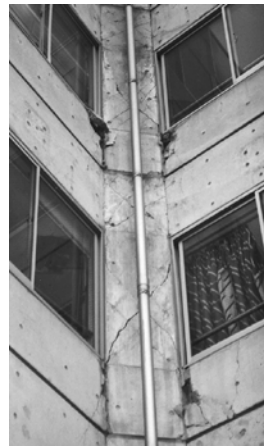
(b) Shearing fracture and damage of pillar
