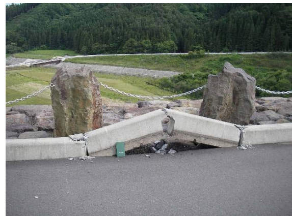
Photo.11 The damaged curbstone on the crest shoulder (Koda Dam) (Photographed by PWRI on June 16, 2008)
