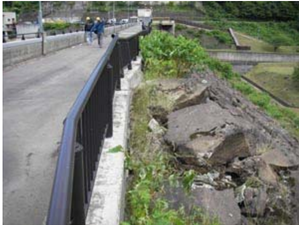
Photo.5 Projection of the riprap rocks around the top of the downstream slope (Ishibuchi Dam) (Photographed by PWRI on June 15, 2008)
