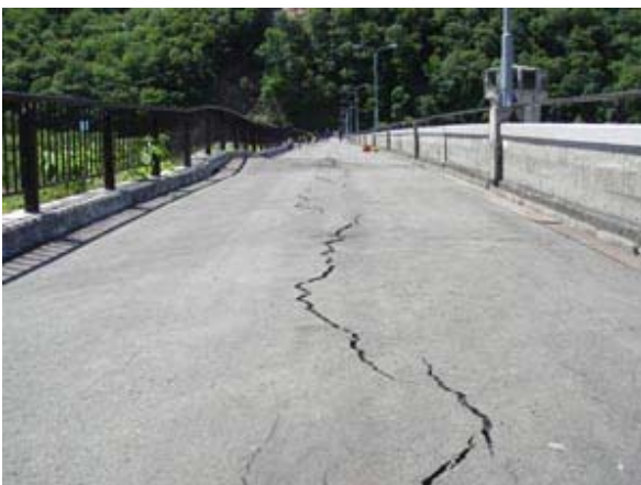
Photo.3 Cracks and waving of the crest pavement (Ishibuchi Dam) (Photographed by PWRI on June 15, 2008)
