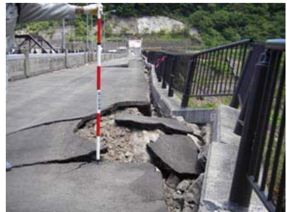
Photo.4 Gaps between the railing and pavement on the crest (Ishibuchi Dam) (Photographed by PWRI on June 15, 2008)
