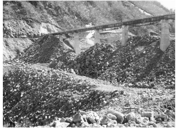
Photo.6 Ishibuchi Dam under construction by the dumped rock method in 1950's (The piers of tramway were buried.) (Courtesy by Kitakami River Integrated Dam Management Office, MLIT)
