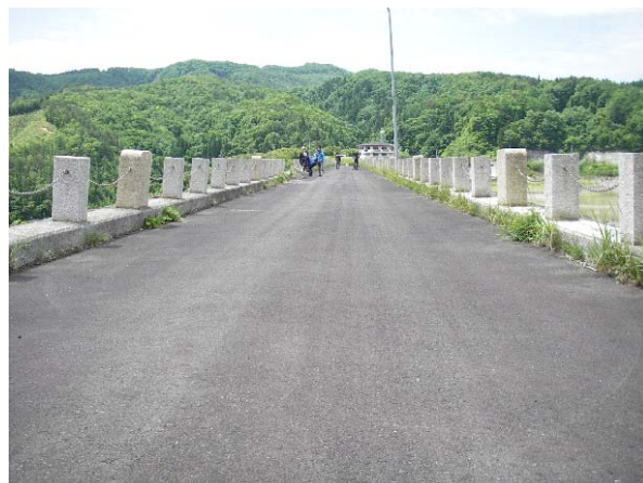
Photo.9 Few cracks in the crest pavement in spite of the dam body settlement (Aratozawa Dam) (Photographed by PWRI on June 16, 2008)
