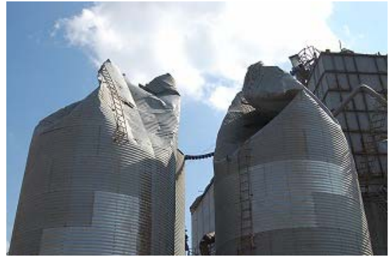
Photo 19 Severe buckling of the cylindrical shells
