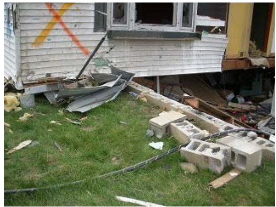
Photo 28 Collapse of continuous footing
