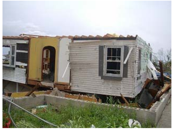
Photo 27 Lateral shifting of entire house
