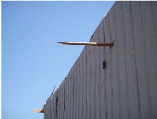
Photo 17 Flying debris impact on the west wall
