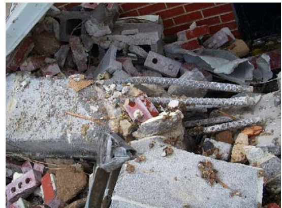
Photo 5 Failure of structural elements reinforced with bars
