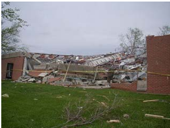
Photo 2 Collapse of wall and roof of classroom
