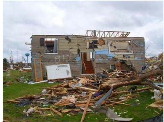
Photo 22 Complete loss of roof
