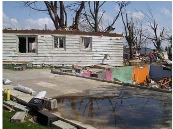
Photo 29 Lateral shifting of entire house
