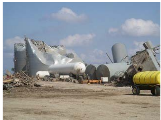
Photo 20 Overturning of smaller tanks
