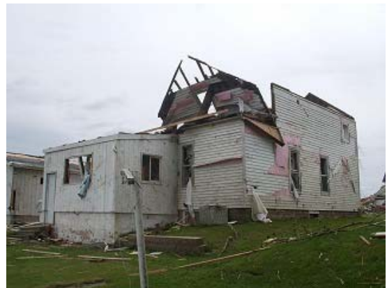
Photo 23 Loss of roof and overturn of the wall
