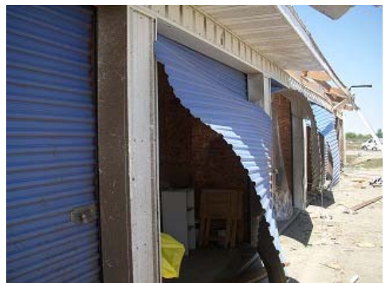
Photo 14 Pulled-out shutters
