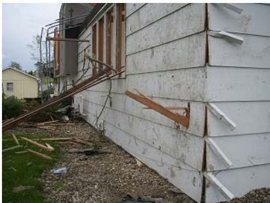
Photo 32 Damage of wall by wind-borne debris impact
