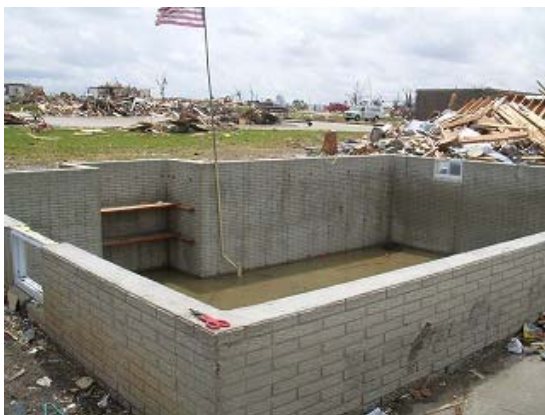
Photo 31 Loss of entire house and swept-clean floor slab
