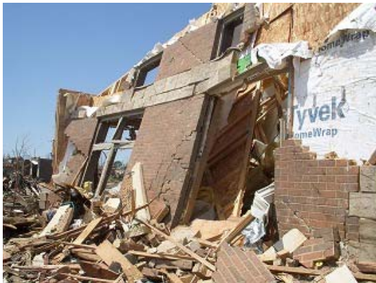
Photo 7 View of south west corner showing collapse of a portion of south wall (Bank A)
