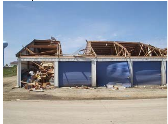
Photo 13 Damaged shutters and roof frames
