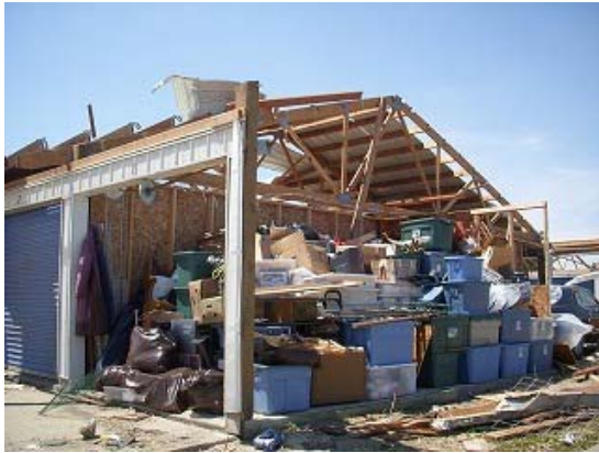
Photo 15 Loss of roof truss and wall
