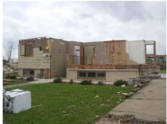
Photo 24 Partial loss of walls
