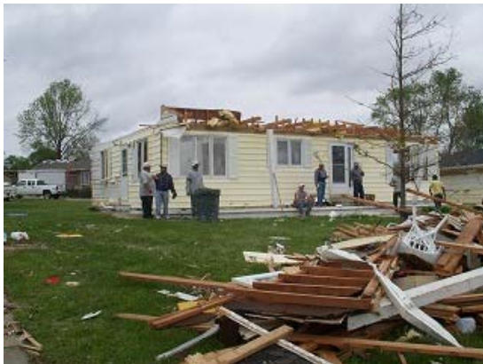
Photo 21 Complete loss of the roof
