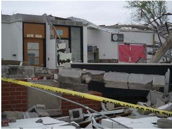
Photo 1 Collapse of wall of classroom
