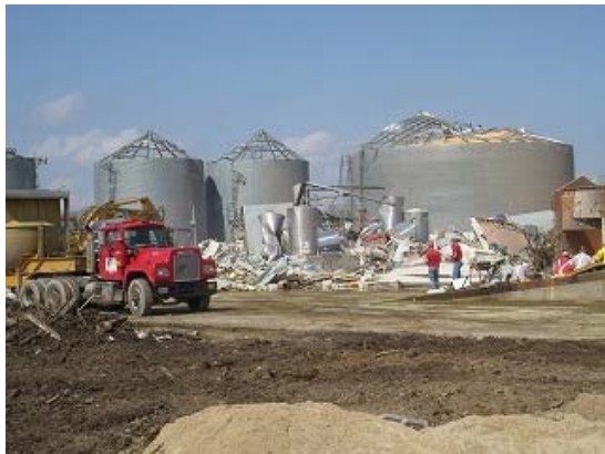
Photo 18 Loss of dome-shaped roof
