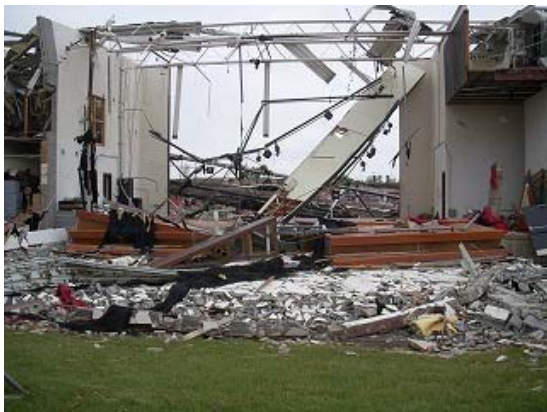
Photo 3 Collapse of wall and roof
