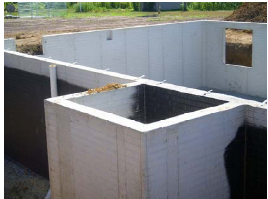
Photo 35 New construction of continuous footing and basement
