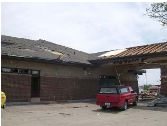
Photo 8 Damage to roof canopy (Bank B)
