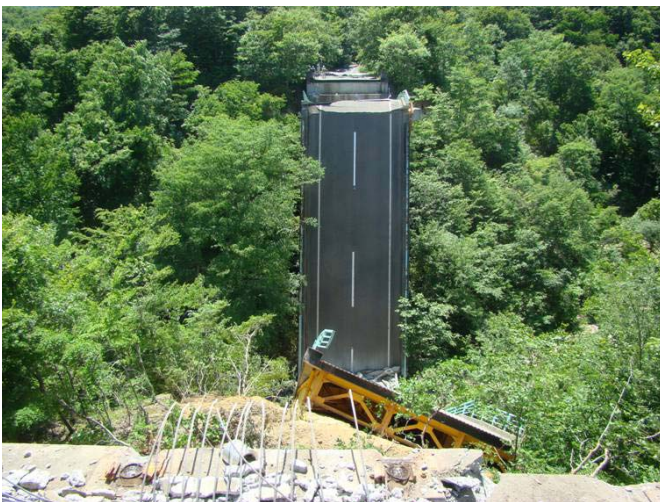
Photo 2 Collapse of Superstructure
