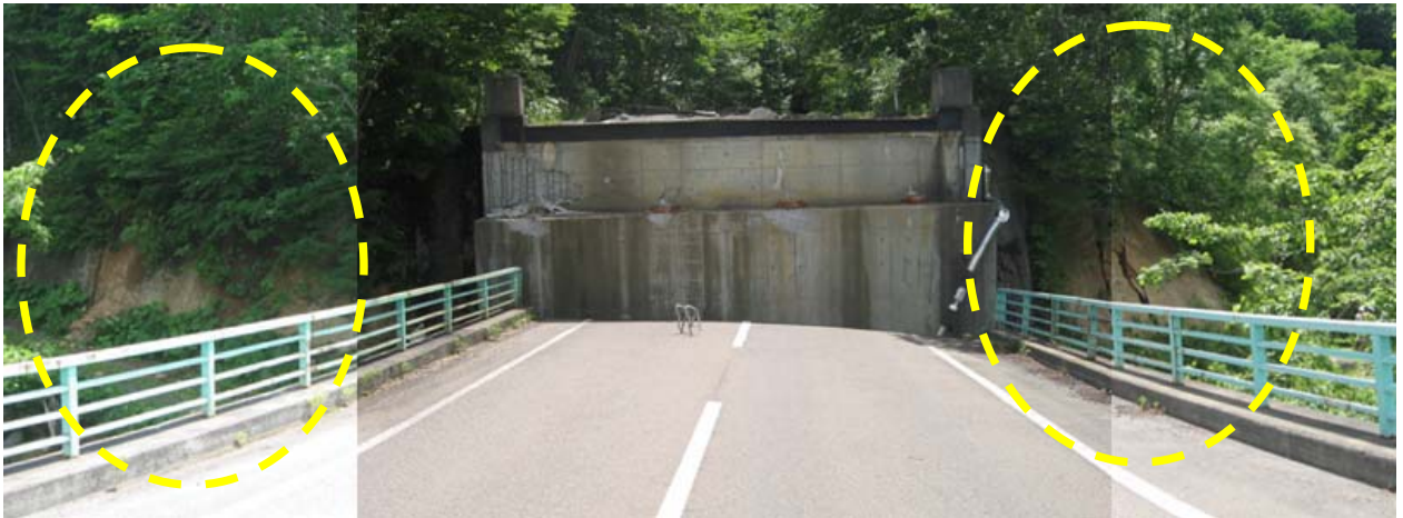
Photo 5 Crack at Slopes in the Back of A1 Abutment
