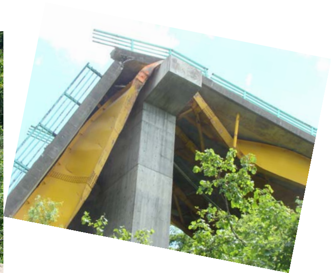
Photo 3 Damage of Girder on P1 Pier
