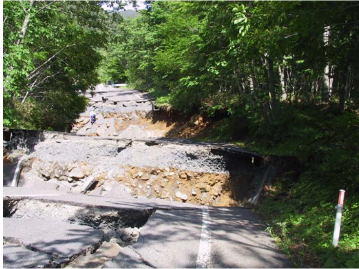
Photo 4 Large Cracks and Slips of Backfill Soils at A1 Abutment
