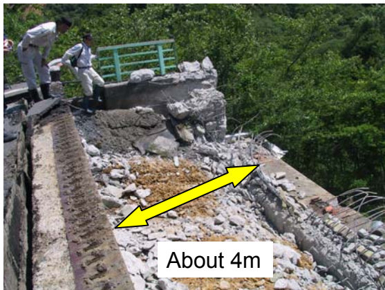
Photo 7 Damage of P2 Pier
