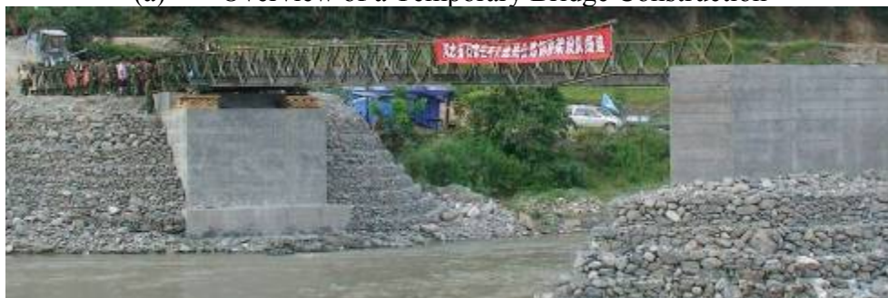
(b) Bailey Bridge Pushed in Place
