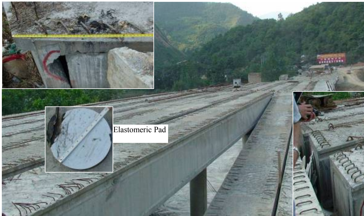
Figure 8: Damage to the 10-Span Bridge under Construction
