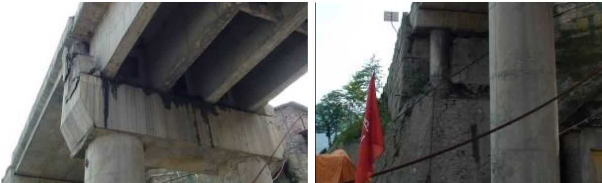
Figure 17: Damage to Shear Key and Embankment of the Overpass
