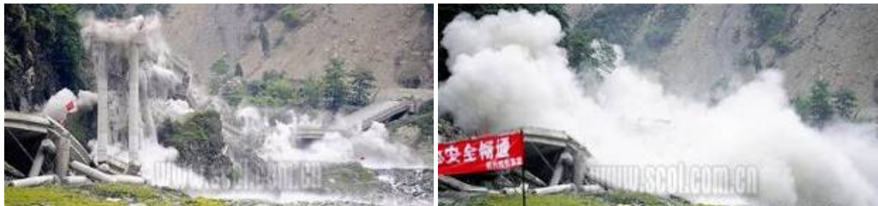
(a) Blast Demolition
