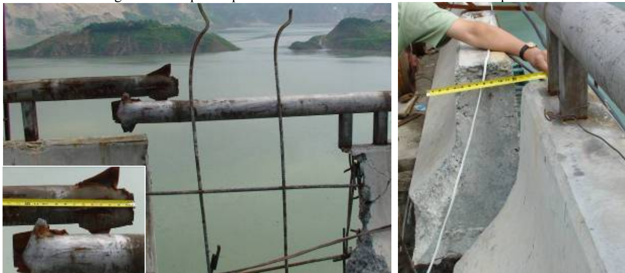
Figure 14: Longitudinal and Transverse Offset of Bridge Deck
