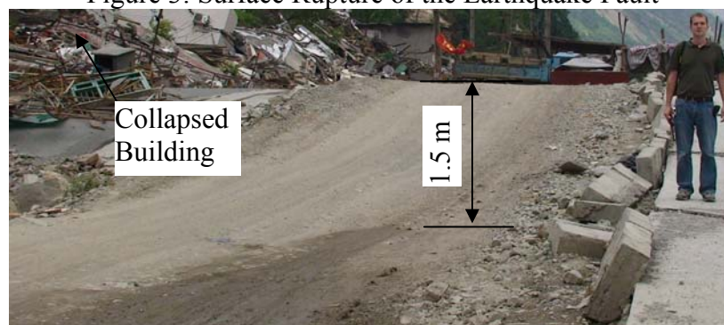
Figure 4: Surface Rupture along the Old Highway near the Collapsed Building
