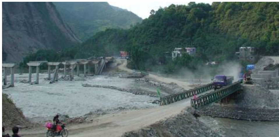
(a) Overview of a Temporary Bridge Construction
