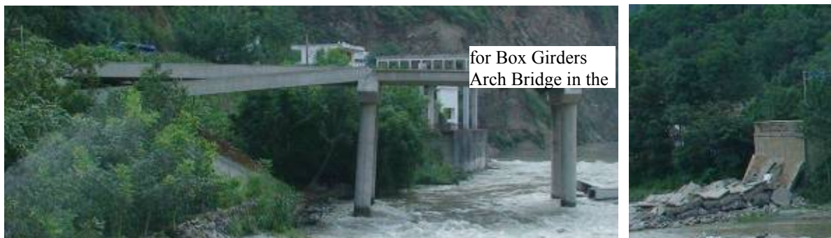
Figure 6: Collapse of the Old Three-Arch Bridge
