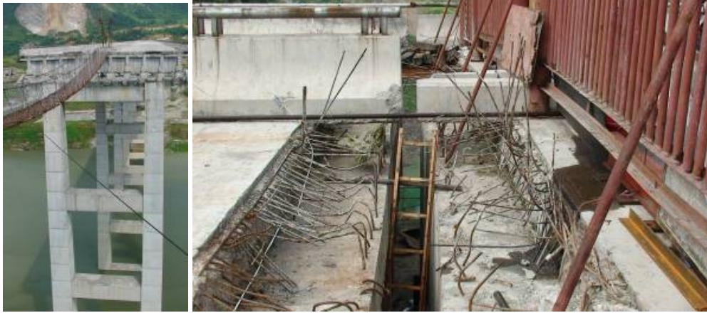
Figure 13: Drop-off Span and Construction Details between Two Spans
