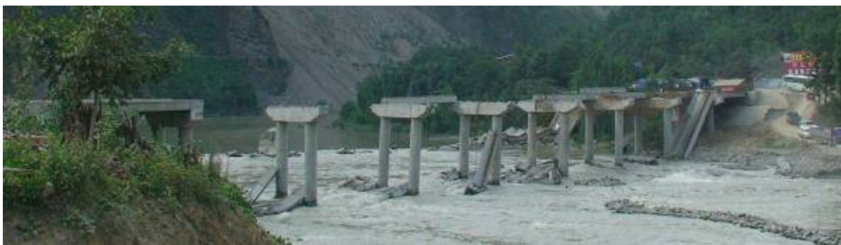
Figure 7: Damage Scenario of the 10-span Bridge under Construction during the Earthquake
