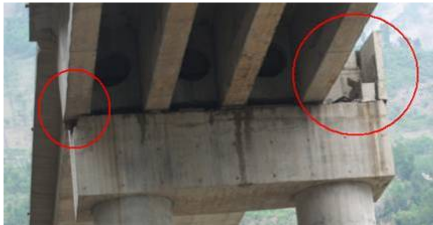
Figure 22: Damage at Bent 9
