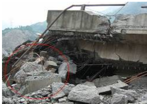
(a) Column Shear and Flexural Failure
