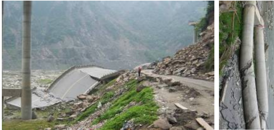
(b) Column Shear Failure and Section 5 Collapse
