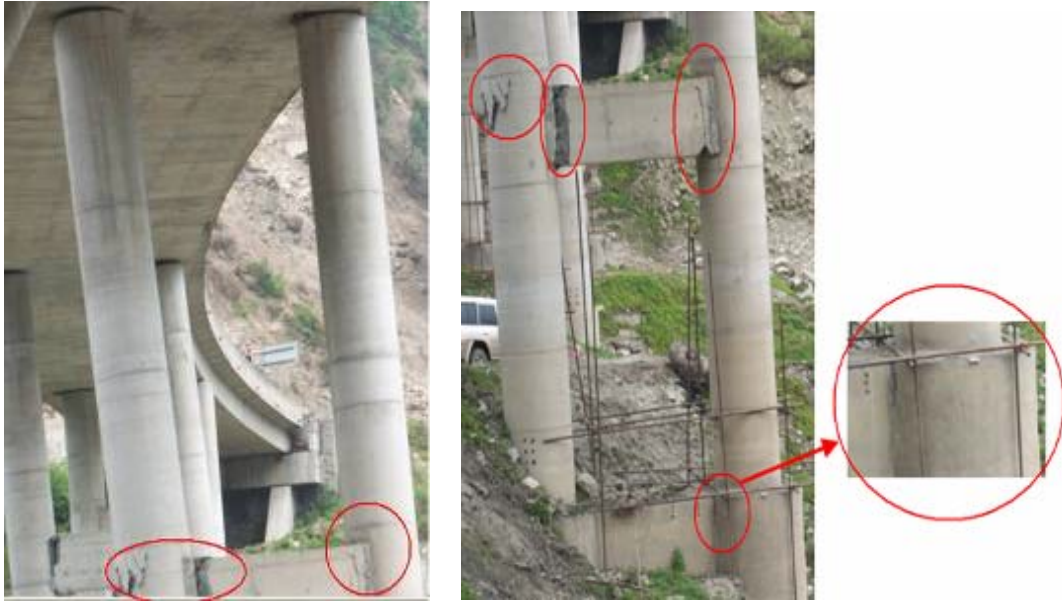
Figure 21: Damage at Bent 3
