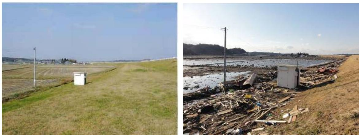
Photo 2 Nakashimo station before (left: 2008) and after (right: April 4, 2011) the earthquake. Tsunami inundation height was about 1m in this area.
