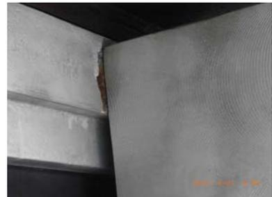
Photo 3 Yamada viaduct and its bearing. The top plates of bearings were scraped by the side blocks.
