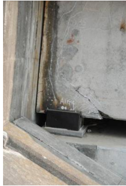
Photo 4 Damage of PC girders near the support
