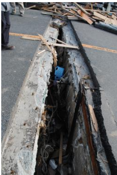
Photo 19 Effective restrainers to tie together adjacent decks
