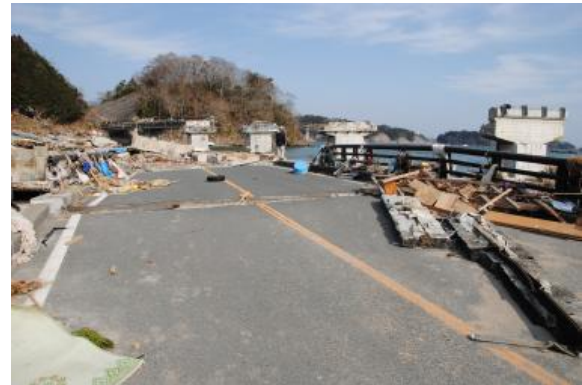
Photo 18 Damage of Utatsu Bridge
