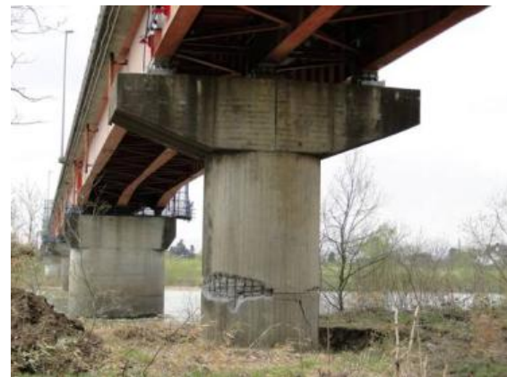
Photo 1 Shear failure of a column due to termination of longitudinal bars with insufficient development (Fuji Bridge) (courtesy of Dr. Hoshikuma, J., PWRI)
