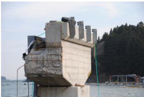
Photo 23 An upper steel bearing after damaged
