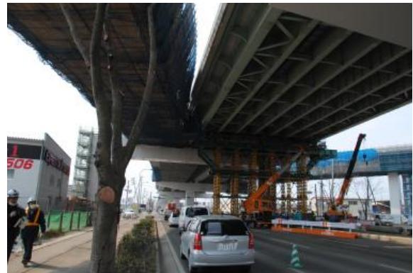
Photo 10 Piers where elastomeric bearings ruptured (Sendai-Tobu viaduct)
