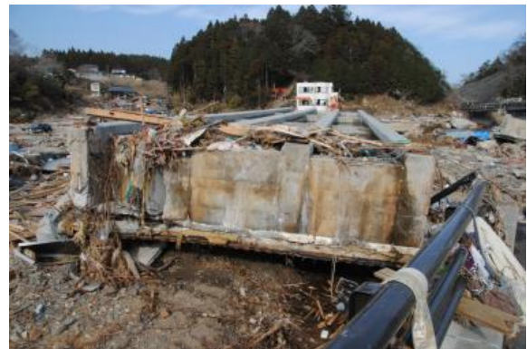
Photo 20 An overturned superstructure
