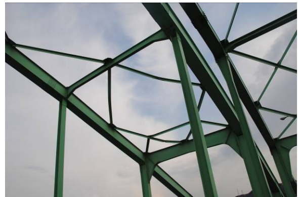
Photo 5 Buckled truss braces
