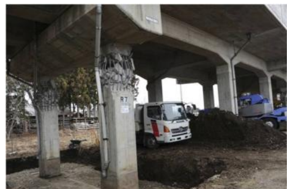
Photo 16 Damage of R7 column, No. 1 Nakasone viaduct during 2011 Great East Japan earthquake
