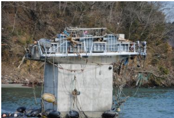
Photo 21 Steel devices for extending seat length (short device) and steel stoppers for preventing excessive longitudinal deck response due to ground motions (tall device)
