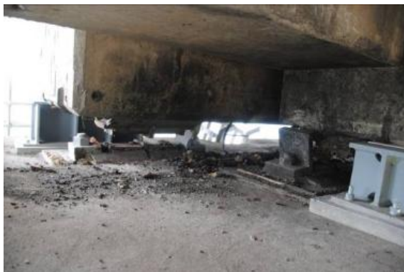
Photo 3 Damage of pin and roller bearings
