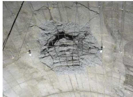
Photo 2: Failure at the Crown of Arch
