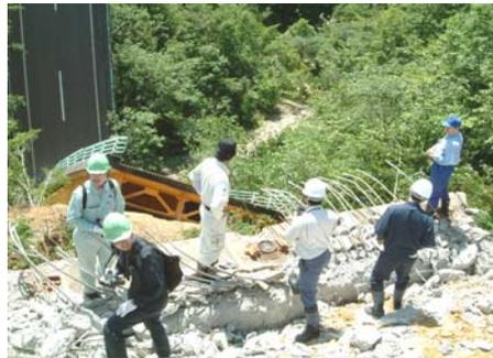
Photo 3. Collapse of Maturube Oh-hashii Bridge during the 2008 Iwate-Miyagi Nairiku Earthquake and emergency scan team by a special unit including CAESAR researchers.
