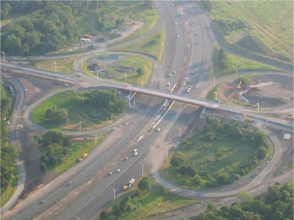
Figure 5 – Ariel view of Scotch Road over Interstate Route 95
