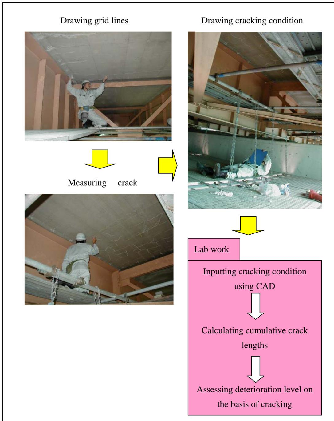
Figure 1 Work Flowchart of Close-range Direct Visual Inspection
