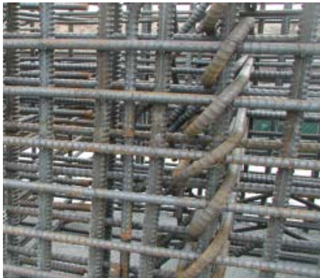
Photo-1 Example of arrangement of reinforcing bar
