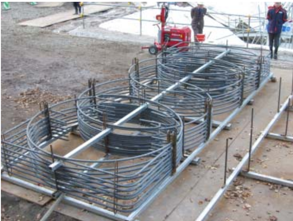
Photo-2 Construction status (1)
