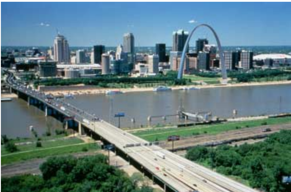
Figure 1. Poplar Street Bridge in St. Louis, Missouri
