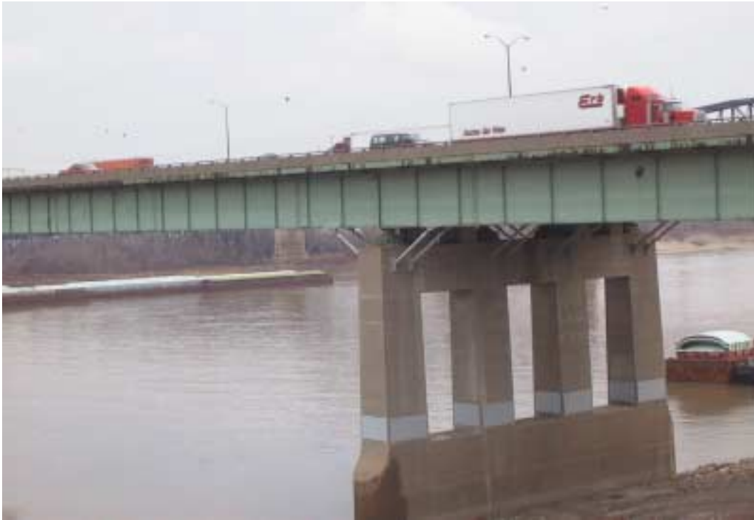
Figure 2. Pier 2 with retrofit installed
