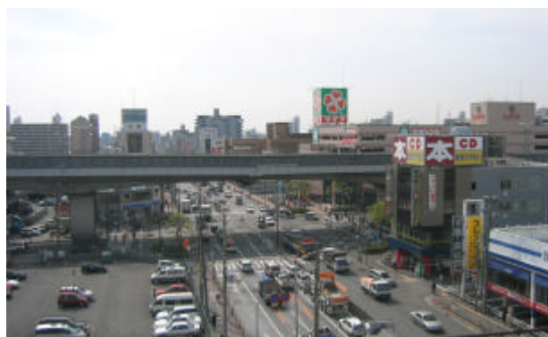
Photo.1 View of the entire Kireuriwari Viaduct
