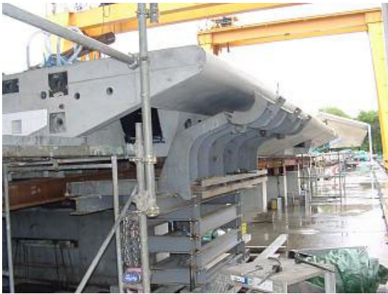
Photo 2 Fabrication of concrete segments
