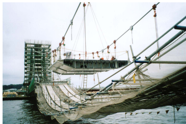
Photo 5 Erection of steel girders
