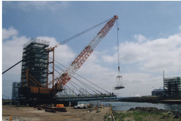
Photo 4 Erection of concrete segments
