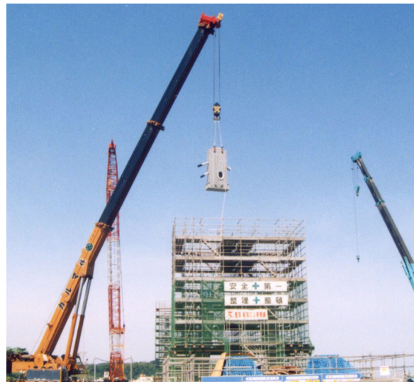
Photo 3 Steel shell member of P2
