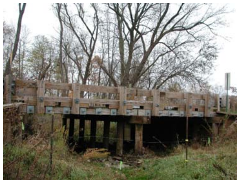
Figure 2—Stress-laminated deck treated with ACQ preservatives.
