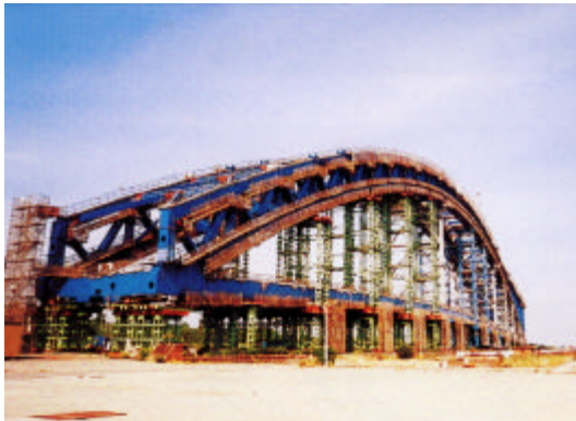
Photo.2 Assembly of Arch Block in the Yard
