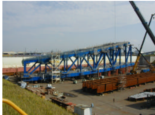
Photo.3 Assembly of Truss Block in the Yard
