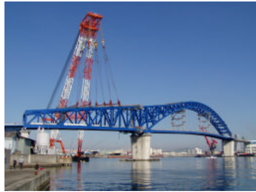
Photo.7 Erection of Truss Block and Moment Joint
