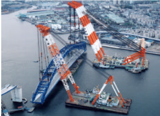
Photo. 6 Erection of Arch Block
