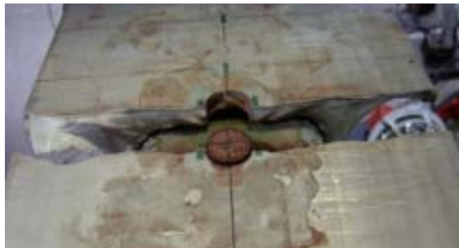
Figure 18. Fatigue crack initiated at the air-release hole of the top flange of the aluminum beam
