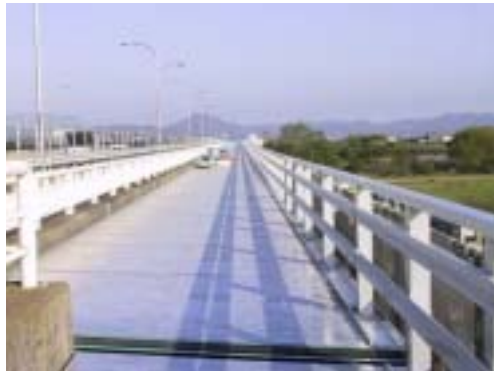
Figure 1. Aluminum deck of the Shin-kakogawa bridge
