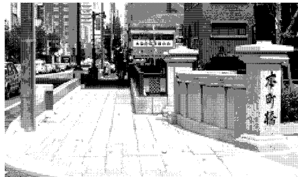
Figure 4. Bridge face of Honmachi Bridge
