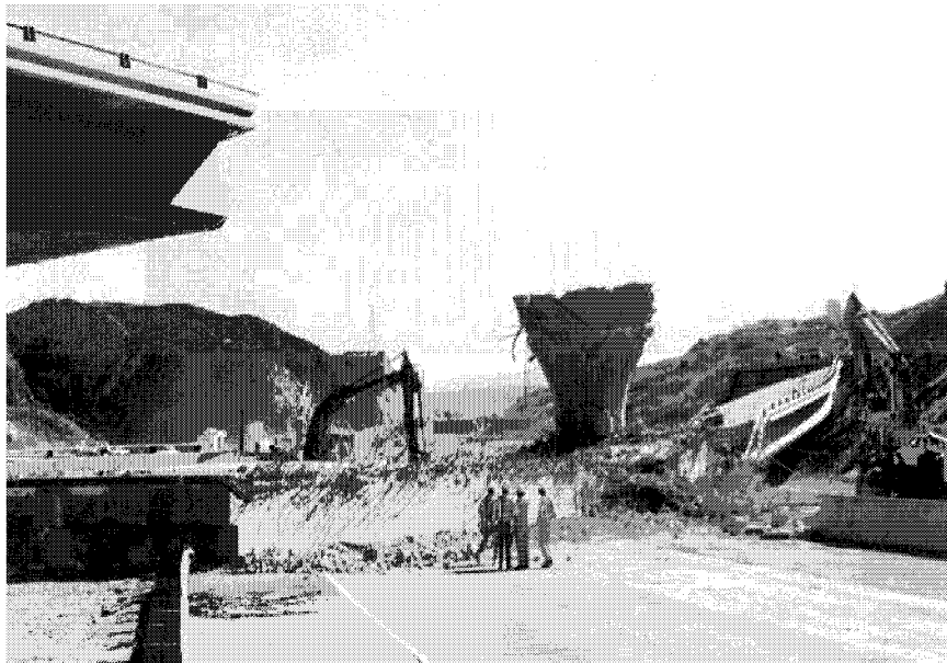
Figure 5 – Damage from the 1994 Northridge Earthquake
