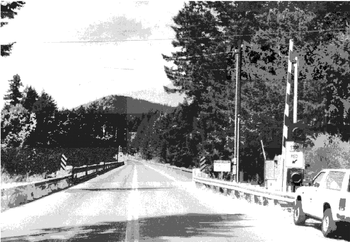
Figure 10 Seismic Gates at the Cedar Creek Bridge
