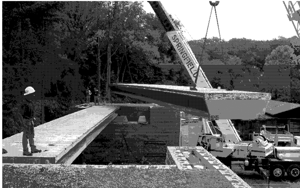
Figure 4. Girder Placement.
