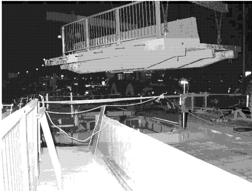
**Figure 4. Prefabricated Deck Panel (Source : [www.pjcci.ca](http://www.pjcci.ca) )**
