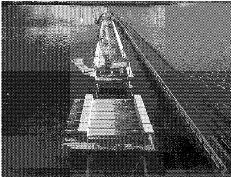
**Figure 10. Installation of Channel Segments of Sorell Causeway Bridge (source: Gibbens and Smith 2003)**
