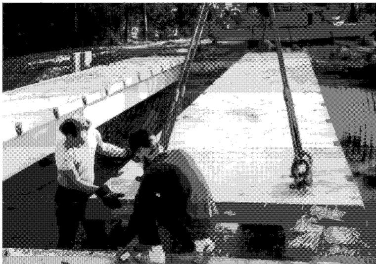
**Figure 8. Double-Tee Bridge System**
