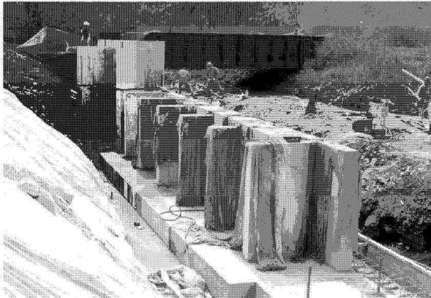
Figure 18. View of Counterfort Abutment System (Source: Scanlon et al. 2002)
