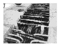
Prefabricated deck systems require that longitudinal and transverse joints be provided to make the deck continuous for live load distribution and seismic resistance. This is accomplished by using special loop bar reinforcement details in the joints. Various joint details observed during the tour should be developed for use in the United States to facilitate the use of prefabricated full depth deck systems.
