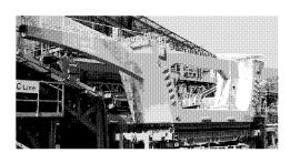
To reduce the weight of precast concrete segments, the Japanese use a segment in which the traditional top slab is replaced with a transverse prestressed concrete rib. After erection of the segments, precast, prestressed concrete panels are placed longitudinally between the transverse ribs. After a topping is cast on top of the panels, the deck is post-tensioned transversely.
