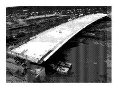
In Europe, it was observed that large bridge components or even complete bridges weighing several thousand metric tons have been built at one location and then lifted and transported to their final location using a series of vehicles known as self propelled modular transporters (SPMTs). These multi-axle computer-controlled vehicles have the capability of moving in any horizontal direction with equal axle loads while maintaining a horizontal load with undeformed or undistorted geometry.
