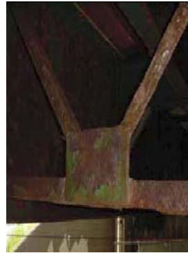
(b)girder and bracing
