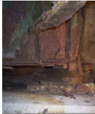
(a)end of girder
