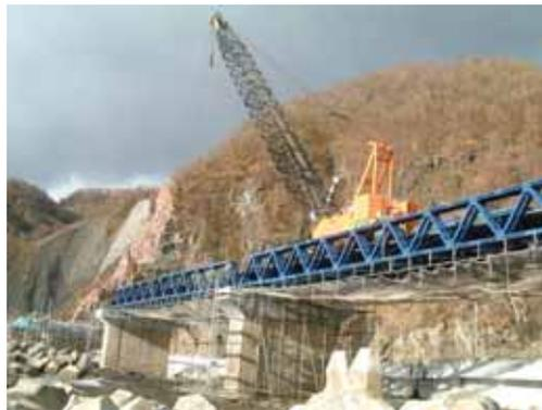
Photo 6: Construction of temporary bridge
