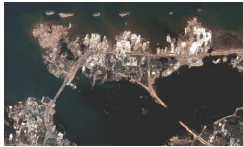
Figure 1b. Damaged Coastline and Bridge Structures, Banda Aceh, Indonesia, after Dec. 2004.
