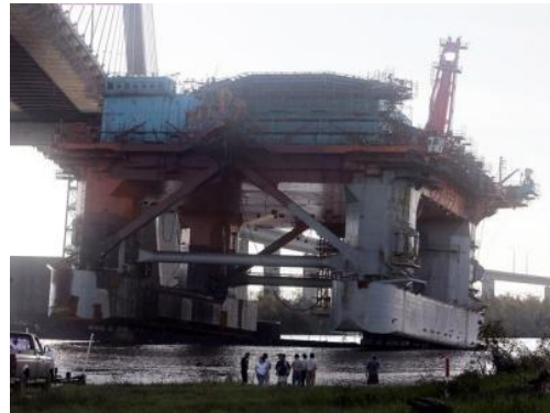
Figure 5b. Oil drilling rig broken loose and hitting the Cochrane-Africatown bridge across the Mobile River in AL during the Sept. 2005 Katrina Hurricane and Storm Surge.
