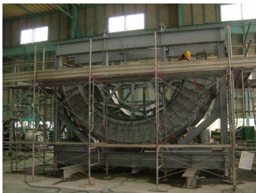
Photo.17 Assembling of the form
