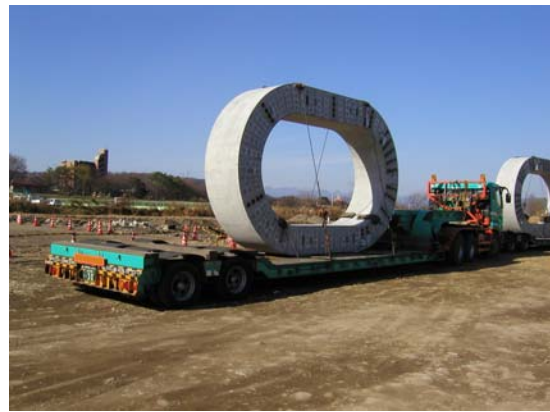
Photo.2 Transport form the factory to the site by trailer
