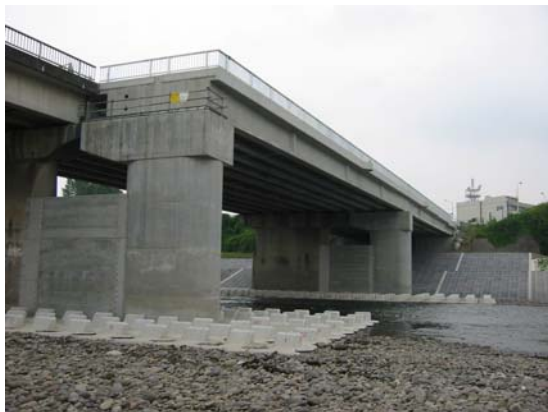
Photo.1 Bridge pier and caisson of the PCa segmental method
