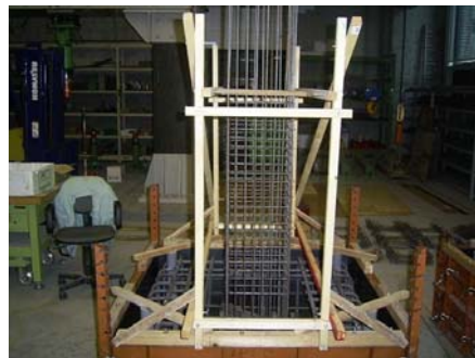
Photo.6 Arranged reinforcing bars
