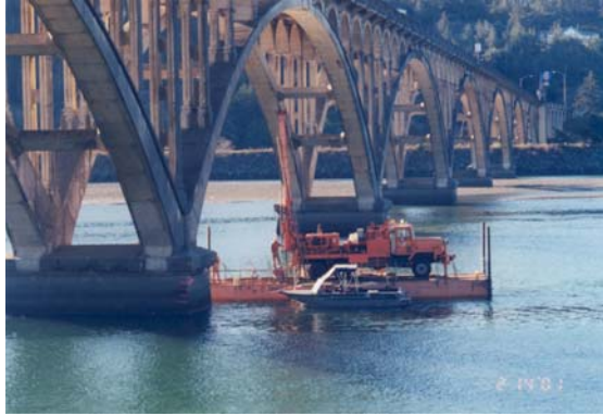
Photo 4 – Drilling subsurface borings at Pier 2.
