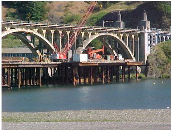
Photo 5 – Pier 2 Drilled Shaft Construction from Temporary Work Bridge
