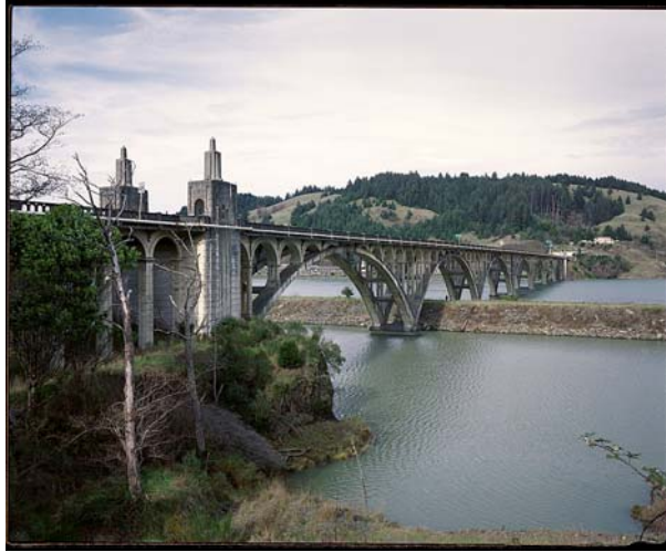
Photo 1 – Rogue River (Gold Beach) Bridge.
