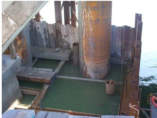
Photo 6 – New footing underpinning has 6- 2.5 m drilled shafts.
