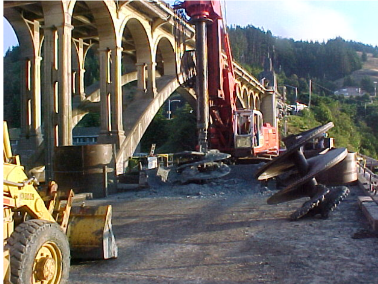
Photo 7 – Drilled shafts were drilled in full length casings 2 m into rock.
