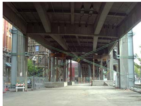
ALASKAN WAY VIADUCT SHORING
