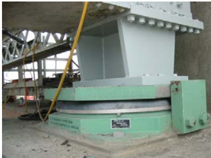
FRICITION PENDULUM BEARING
