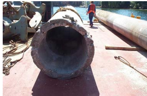
TYPICAL PRESTRESSED CONCRETE HOLLOW COLUMN
