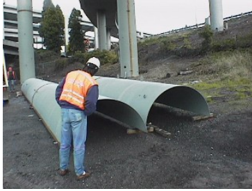
COLUMN RETROFIT STEEL
