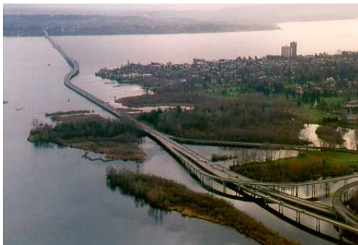
SR520 – EVERGREEN PT FLOATING BRIDGE AND APPROACHES
