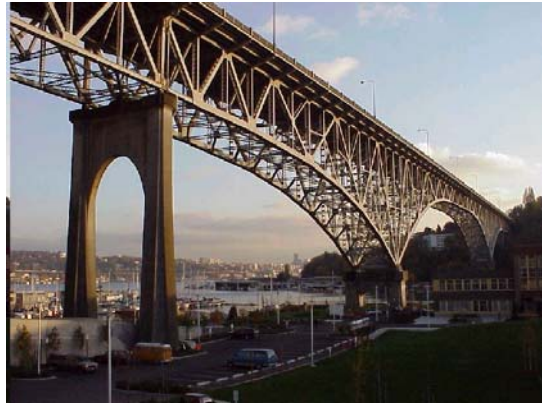
GEORGE WASHINGTON BRIDGE
