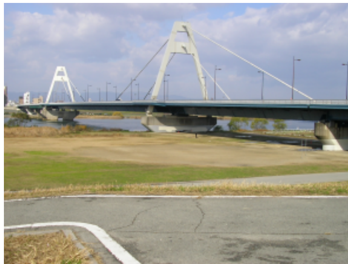
Photo.1 Panorama of Toyosato Bridge
