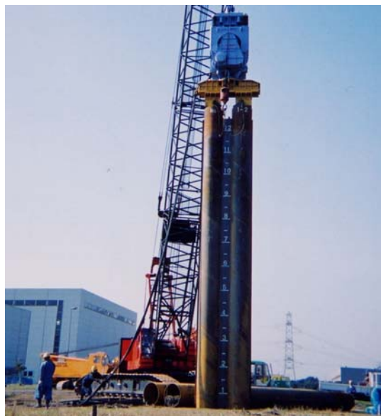
Photo 3. Overall situation regarding the field construction test for H-joint SPSP
