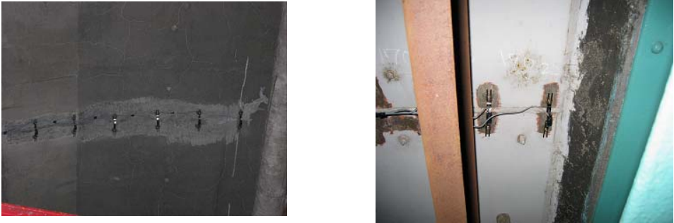
(a) New bridge (b) Old bridge
