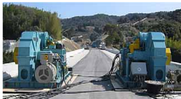
Photo 4 Installation of Exciters
