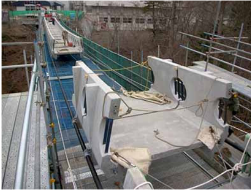
Fig. 17 Erection of Precast Segments
