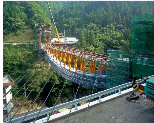
Fig. 11 Side Wire Stabilizers
