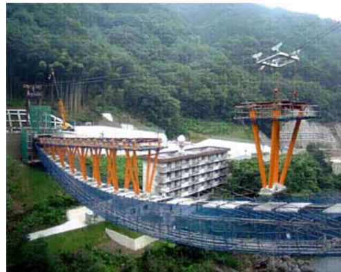
Fig. 9 Erection of Diagonal Unit
