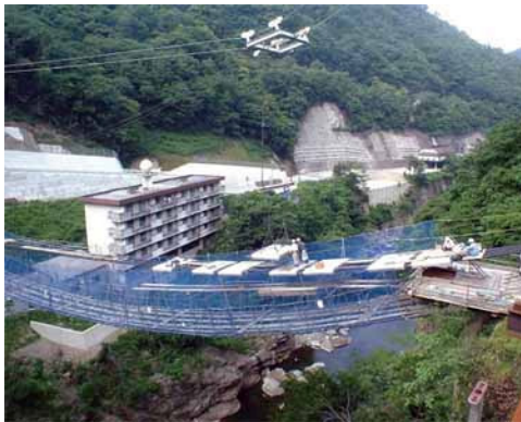
Fig. 8 Erection of Precast Panel
