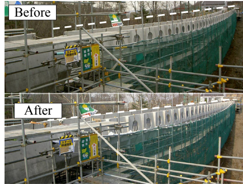
Fig. 18 Adjustment of Secondary Cables
