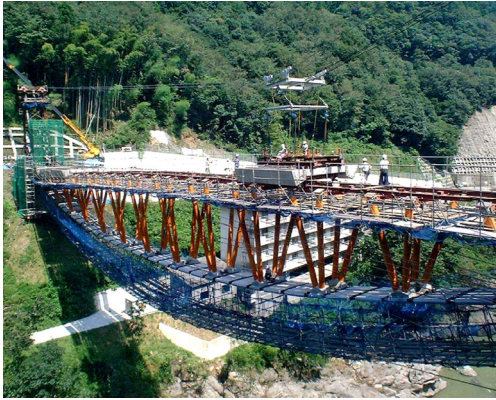
Fig. 10 Erection of Girder Unit
